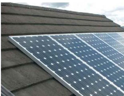
Solar Panel Roof
